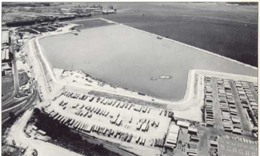
The 146 acre Canton/Seagirt Dredge Disposal Site will hold 3½ million cubic yards of material dredged from the harbor bottom. It is anticipated that the site will be converted by others into a marine terminal in the future.
